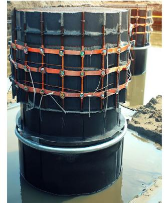
image: Pile head protection system
